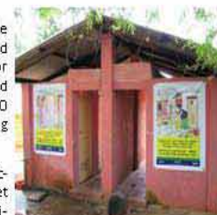
Rehabilitated toilets with Hygiene messages
